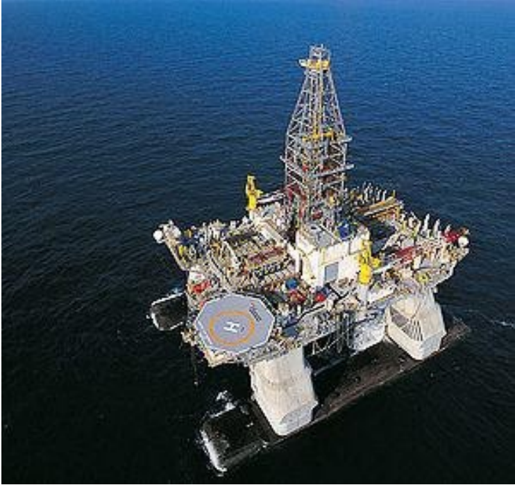
Figure E.15. Deepwater Horizon mobile offshore drilling unit. Image: Transocean
